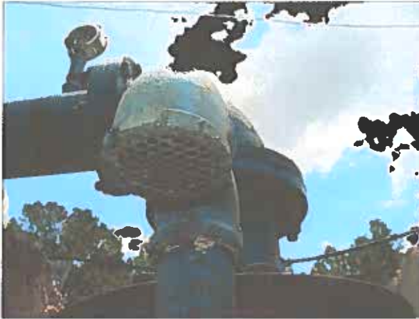
Attachment #21 Severity: Minor Facility ID: WELL 4 SOUTH Category: Source Attachment Comments: Well vent screen not #4 Stainless steel mesh
