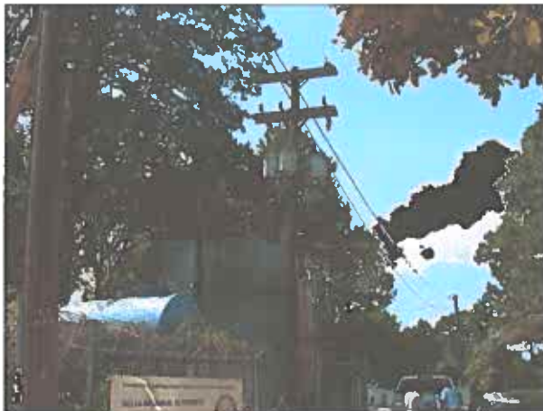
Attachment #24 Severity: Significant Facility ID: GROUND 1 NORTH Category: Finished Water Storage Attachment Comments: Tree limbs hanging over and touching the roof of ground storage tank #1 north
