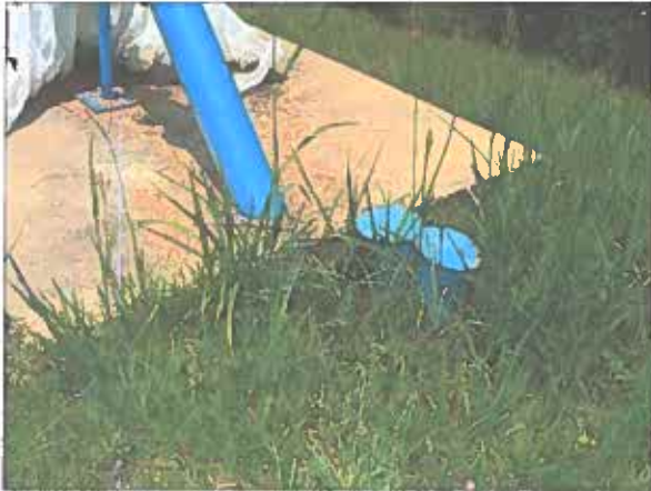
Attachment #5 Severity: Significant Facility ID: WELL 3 NORTH Category: Source Attachment Comments: Well#3 North well slab erosion - picture #2
