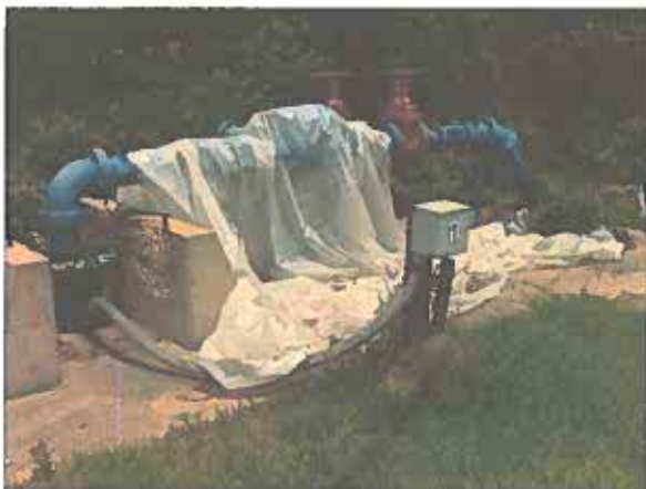
Attachment #7 Severity: Significant Facility ID: WELL 4 SOUTH Category: Source Attachment Comments: Well#4 South well slab erosion - picture #1
