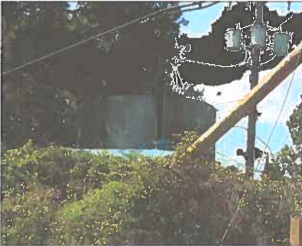
Attachment #23 Severity: Significant Facility ID: GROUND 1 NORTH Category: Finished Water Storage Attachment Comments: Tree limbs hanging over and touching the roof of ground storage tank #1 north
