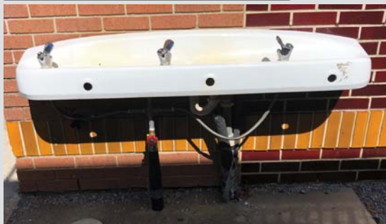
DF10 – BUBBLER OUTSIDE NEAR 5 TH GRADE PLAYGROUND 3 SPOUTS, GOOD FLOW
