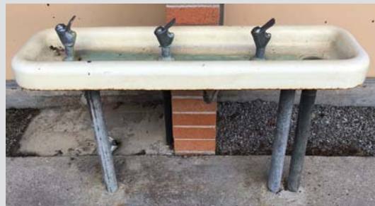
DF11 – BUBBLER OUTSIDE IN SPECIAL SERVICES PLAYGROUND VALVED OFF, BUT FLOWS WHEN VALVE OPENED
