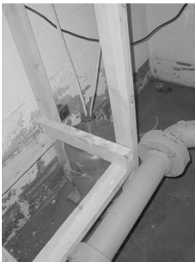
Improper Chlorine day tank
