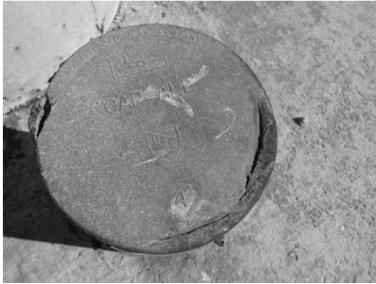
Cap to casing fill tube cracked
