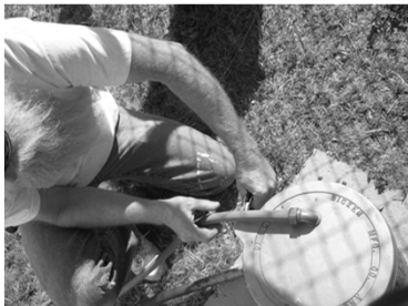
Not a potable water cap (no seal, no vent)
