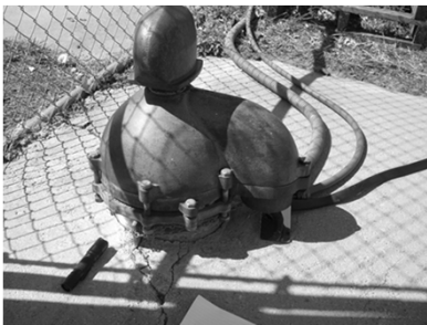
Pitless adapter with low casing, cracked pad
