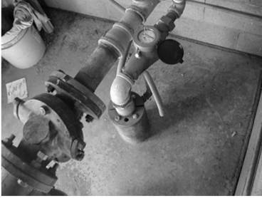
Hole in casing seal
