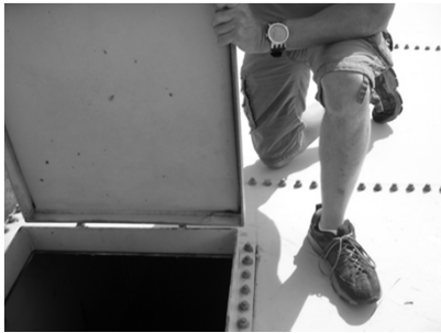
Hatch has no gasket to create seal
