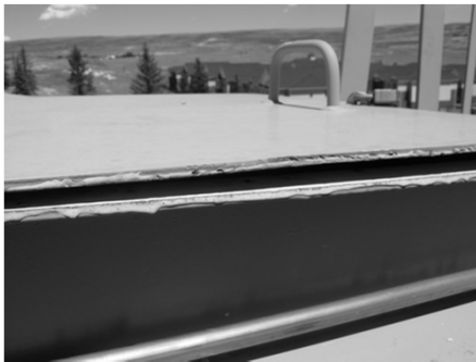
Flat hatch (not knife edge) without seal
