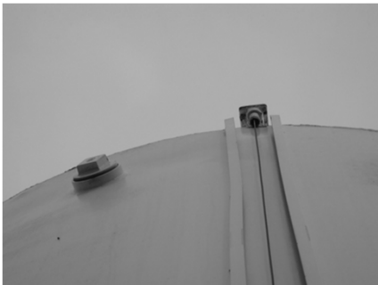
Bad seal on water level indicator, No overflow
