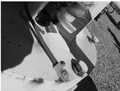
Bolts for well head seal not tight, Vent too low, screen too large
