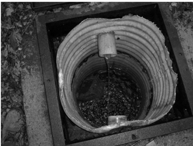
Spring Box - seal missing
