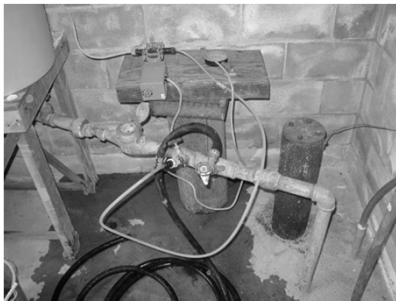
Chlorine pump is unsecured, portable cross connection
