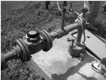
Vent casing is low, not facing down, not 18" off deck
