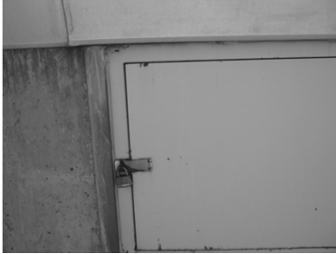
Hatch on side of tank no seal
