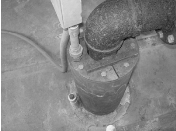
Compression seal that does not seal properly
