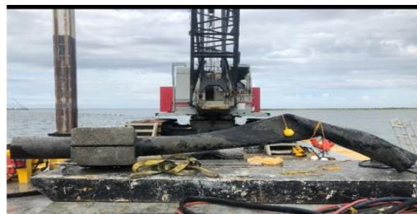
Grand Isle – Transmission pipe wrapped around oil production pipeline
