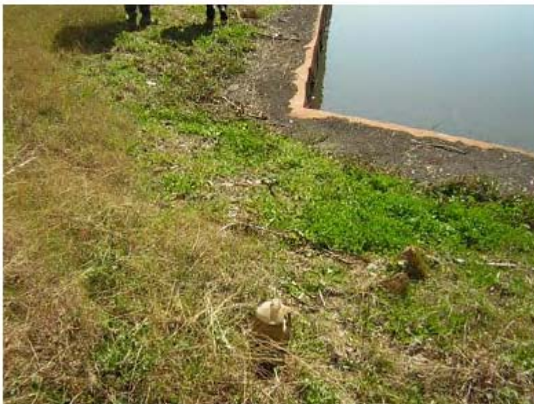
Photo 30: Dried sediment on top of sheet pile wall along bayou and debris left behind by floodwaters associated with Hurricanes Katrina/Rita. Taken 2/16/2006
