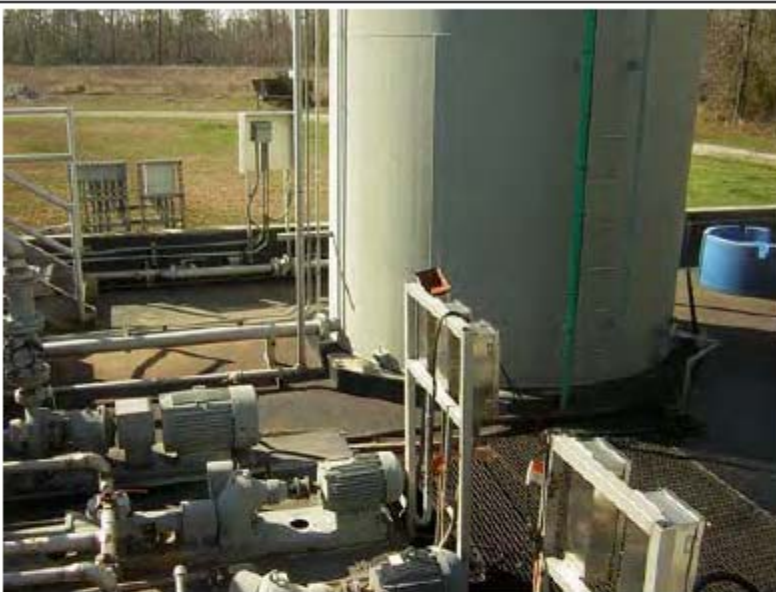
Photo 7: Bottom left, pumps within ground water treatment system, submerged and damaged during Hurricane Katrina. Taken 2/16/2006.
