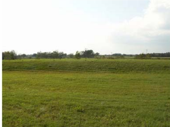
File Name: GSV_photo2.JPG Date/Time Taken: 01 Oct 2005 1631 Description: View to northwest of cap, showing no subsidence, ruts, or cracks due to storm. N29°57'28.1"; W92°11'11.4"
