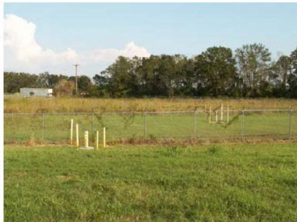
File Name: GSV_photo4.JPG Date/Time Taken: 01 Oct 2005 1641 Description: Boundary fence between Gulf Coast Vacuum and D.L. Mud sites, view to east. N29°57'28.1"; W92°11'11.4"
