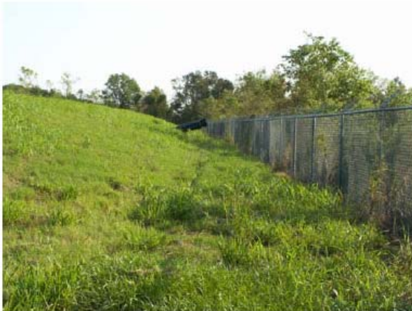
File Name: GSV_photo7.JPG Date/Time Taken: 01 Oct 2005 1652 Description: View to south along western fence and site boundary, showing intact sumps on side of cap. N29°57'31.9"; W92°11'14.1"
