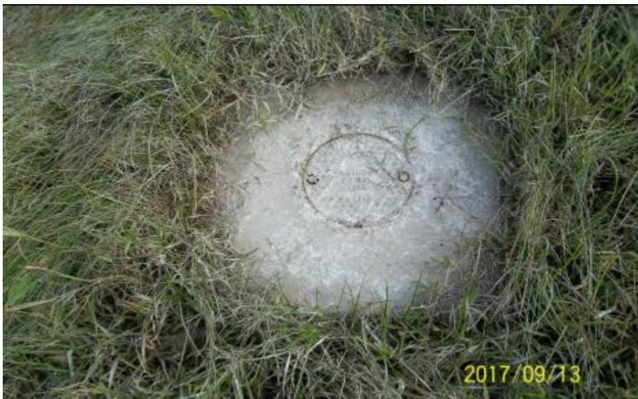
Close view of monitoring well 7 (MW-7) showing the concrete surface completion; location of sample GSU-GW-001.
